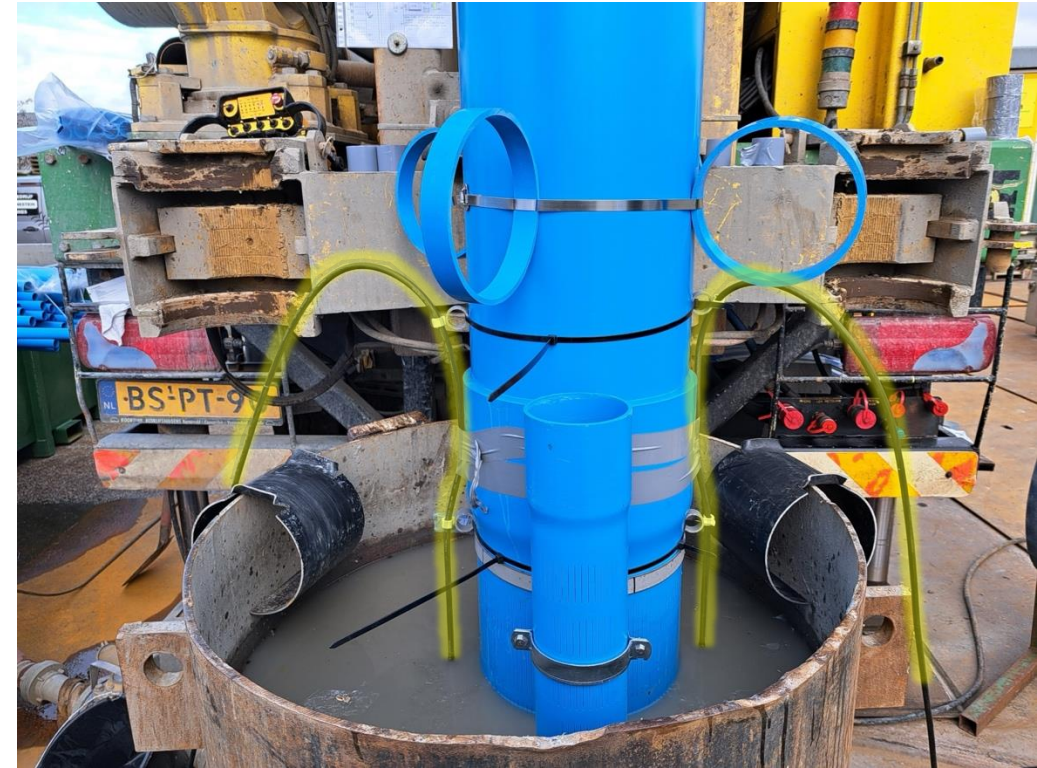
Well screen installation (with FO attached)
